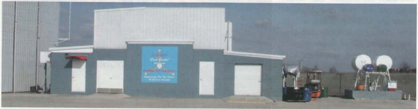
GAMI's aircraft engine test facility and small fuel farm off to the right.
